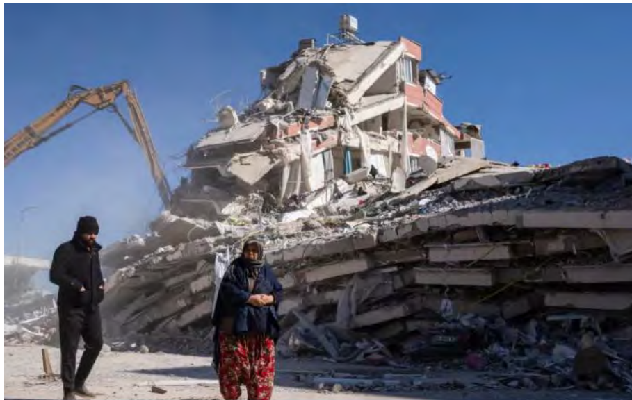
Figure 2: Post-Earthquake Infrastructure Damage in Türkiye (Aljazeera, 2023)
